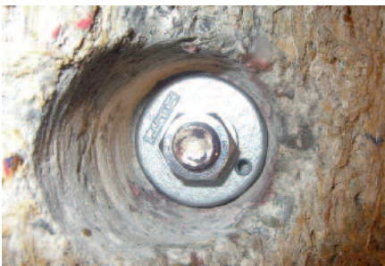
Fig. 8: anchor head
